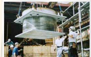
Installation of a 1500mm diameter isolator for High City Kyosumi Condominiums in Japan.
